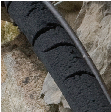
Protect your HVAC foam insulation from harmful UV rays with Dura HVAC Wrap.
